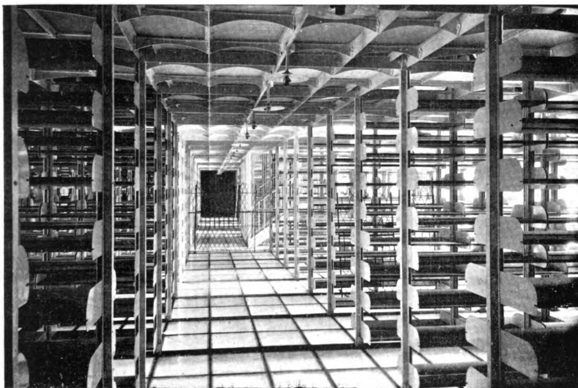
FOURTH FLOOR OF STACK.
