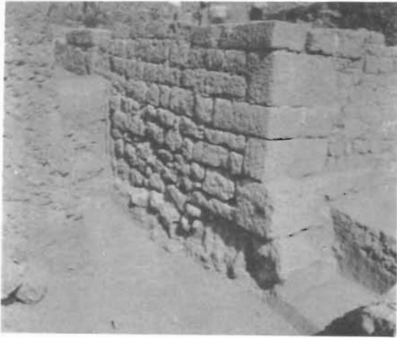
FIG. 18. South market, north wall detail
